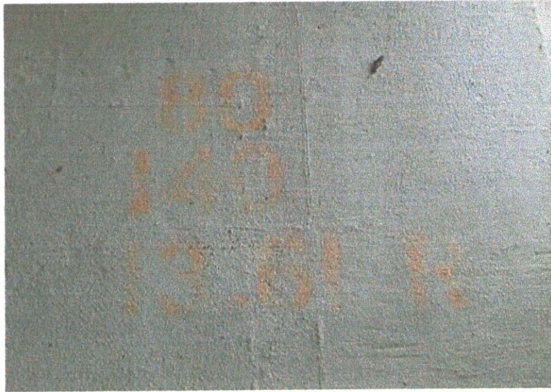
BRIDGE NO. AT ABUTMENT # 1
