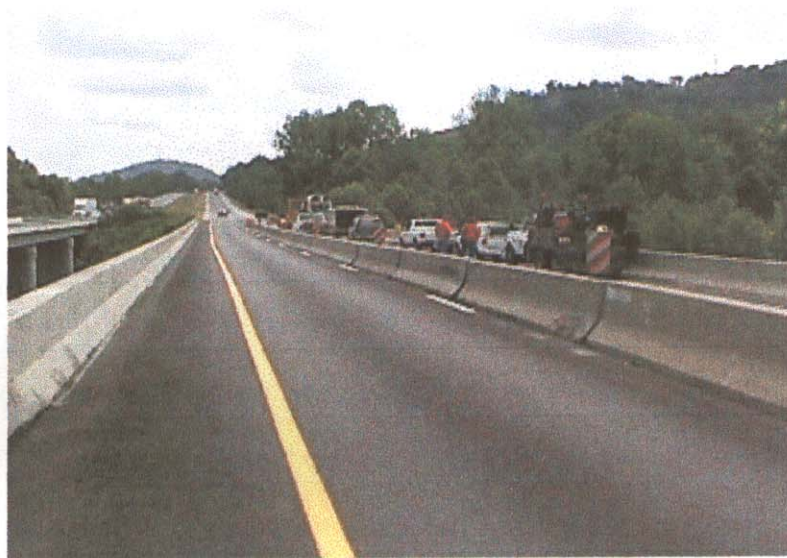
ACROSS TOP OF DECK
