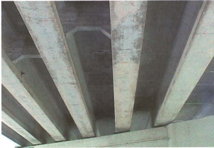
BOTTOM OF DECK
