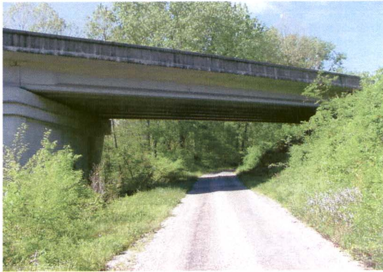
LEFT SIDE VIEW @ UNDERPASS
